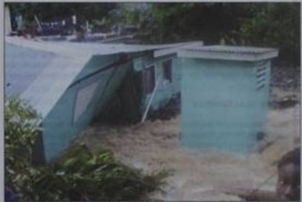
A Massacre house is overwhelmed by the raging flood waters.
