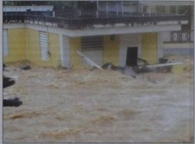
One of several Massacre homes affected by flooding.
