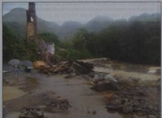
The former Warehouse Disco was destroyed by the heavy flood waters.
