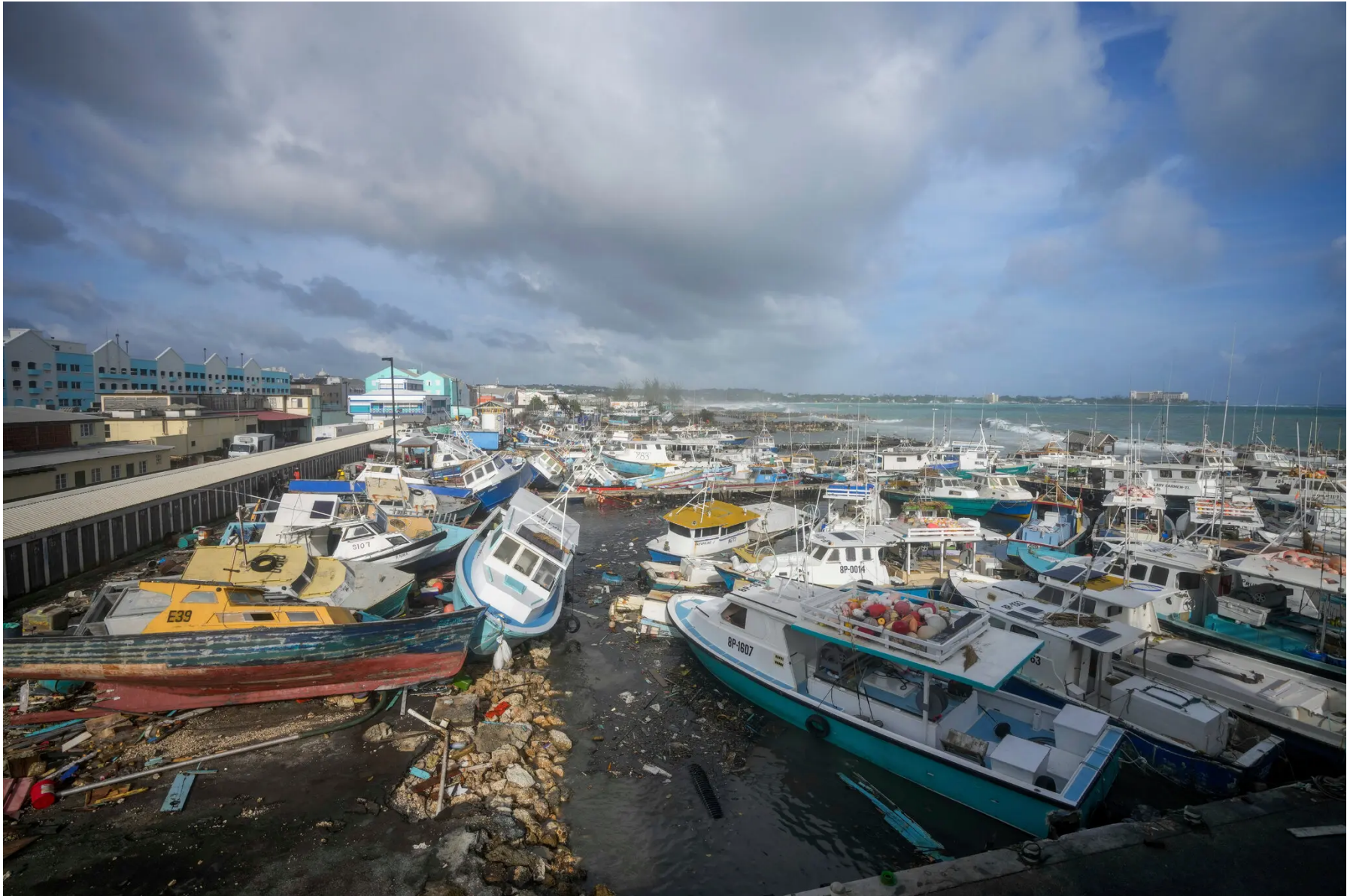
Figure 11. Damaged fishing boats at Bridgetown, Barbados, caused by Hurricane Beryl. Image courtesy of Ricardo Mazalan/Associated Press.
